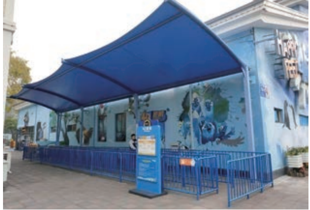
Qingdao Haichang Polar Ocean Park revamped the 4D theater by installing a sunshade 青島海昌極地海洋公園4D影院遮陽棚改造
